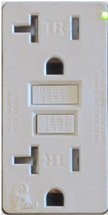
Tamper-resistant (TR) receptacle: TR is molded into the face
