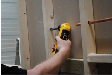
Right-angle drill boring a stud
