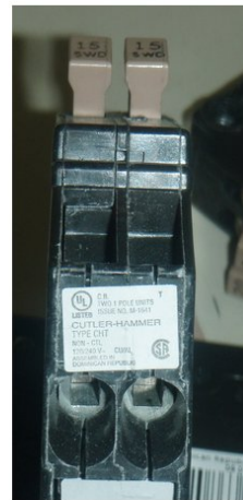
Tandem breaker (two circuits, one space)
