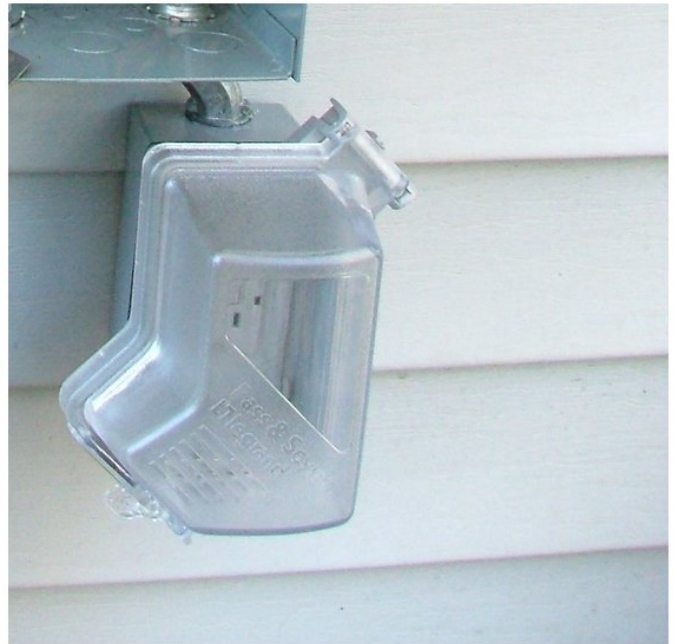
Outdoor box with an in-use (bubble) cover
