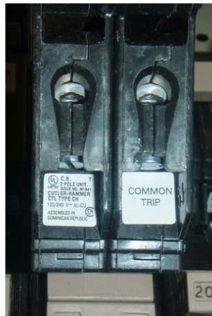
Two-pole breaker (two spaces, common trip)
