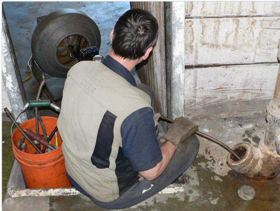
A motorized sewer machine clearing a residential side sewer. The cable runs from the drum into a cast iron cleanout wye at right; spare cutter heads and tools are in the orange bucket.
