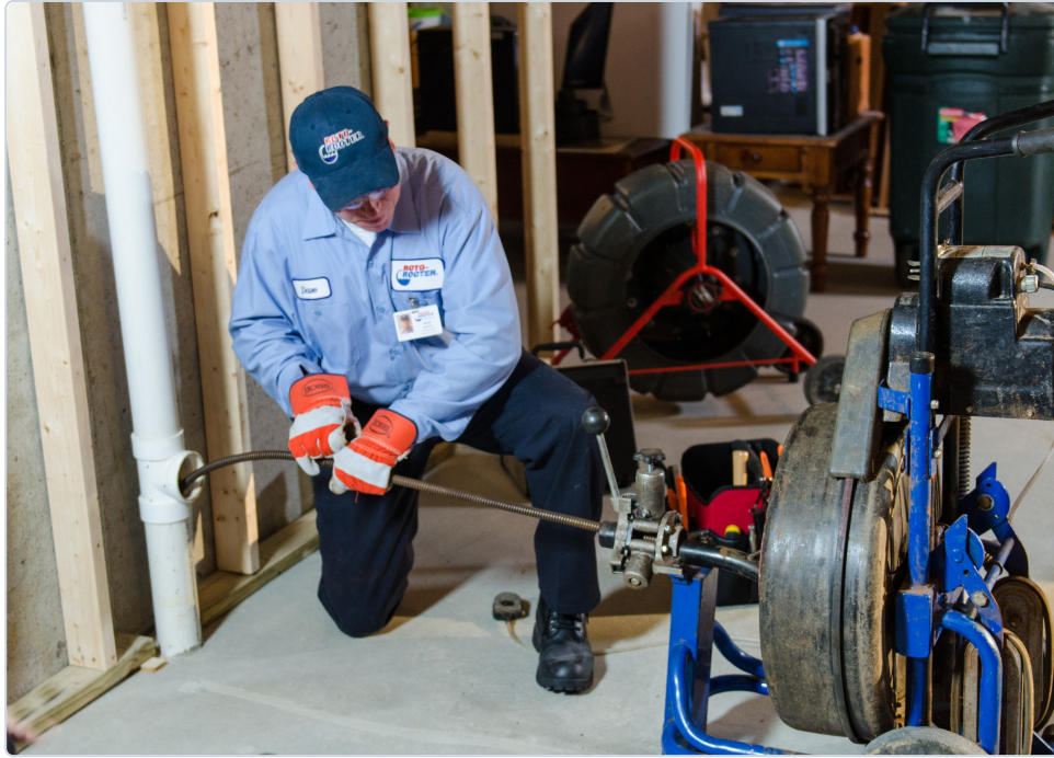
A drum machine (sectional drain cleaner). The technician feeds the steel cable from the rotating drum into a cleanout opening on a PVC stack; the drum spins the cable while he guides it with gloved hands.
